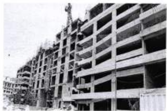
Fig: Construction at the site
